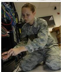
Senior Airman Holly Durkin, a Cyber Surety Technician for the 129th Communications Flight, Moffett Federal Airfield, Calif., replaces an uninteruptable power supply (UPS) from a network server, August 4, 2010. The UPS serves as back-up power supply for network servers in case of main power loss. (Air National Guard photo by Tech. Sgt. Ray Aquino)
